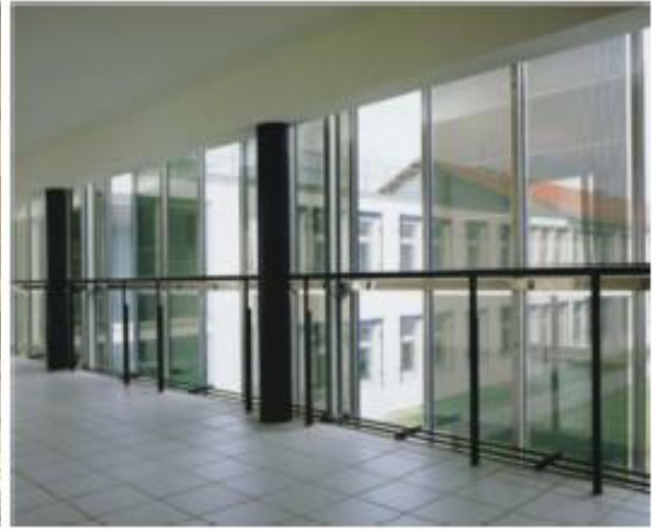
Figure 5: Semi-transparent facade[7]
