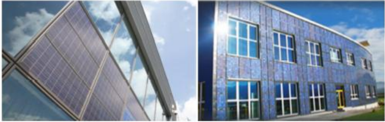
Figure 7: Cladding systems[6]
