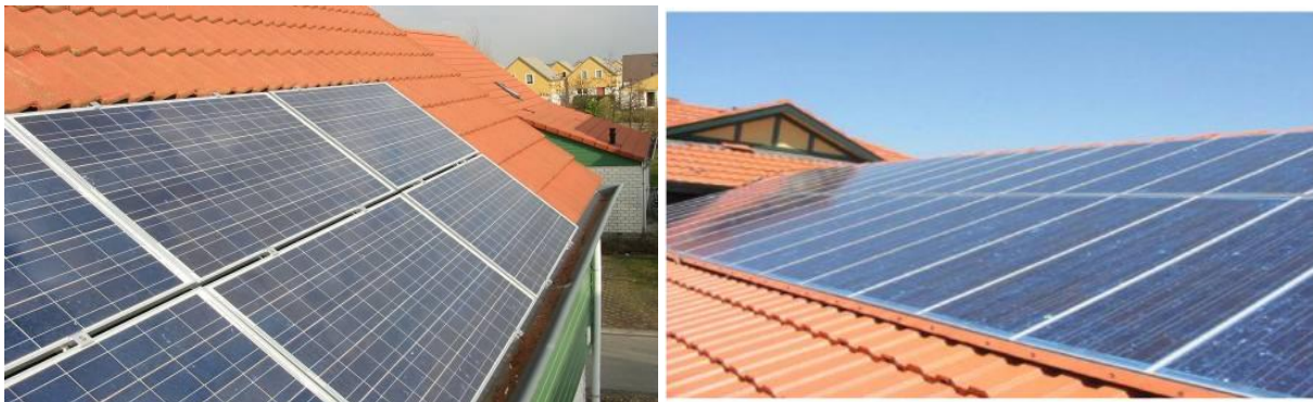
Figure 2: Example of an in-roof PV system.
